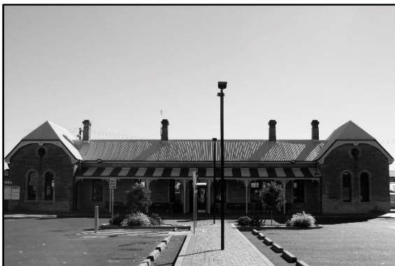
Dubbo Railway Station (opened 1881) 2017 Has changed little since 1916 Author's photograph
